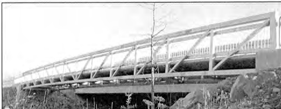
FIGURE 2. An example of the truss type of superstructure to be used for the Bridge No. 6011 replacement. The photo is of a pedestrian bridge in Anchorage over Ship Creek. (The concrete bridge in the background is the Glenn Highway.)
