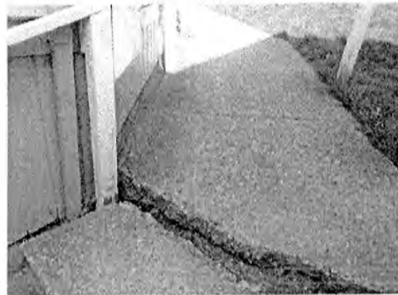
Separation of concrete walkway between structures is a potential tripping hazard.
