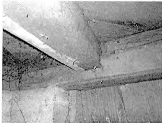
A 2x6 joist has been scabbed onto a 4x6 timber joist to reinforce the rotten ledger connection. (Church Building)
