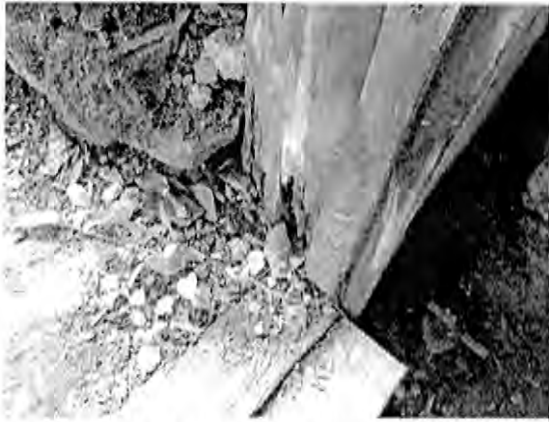
Rotten door jambs at the lowered entries in the rectory indicate poor drainage.
