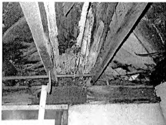
A severely rotted timber floor beam has been reinforced with two 2x6 joists in the basement of the rectory.
