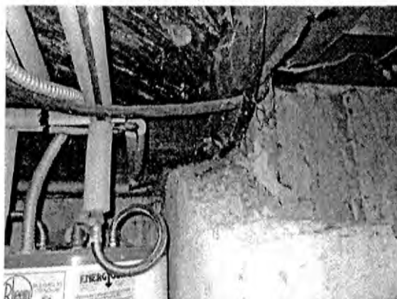
The wood floor above the water heater shows significant signs of water damage, which is reflective of the rotten siding on the exterior of this wall. (Rectory)
