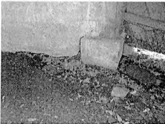
The foundation wall is being undermined near the concrete walkway. Note the downspout to the right. (Church building)
