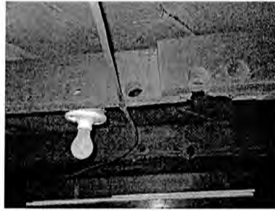
2x6 timber joists on the east side of the rectory have lost most of their strength due to excessive drilling.
