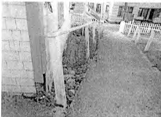
Wood siding and trim is rotten on lower wall of rectory building from standing water.
