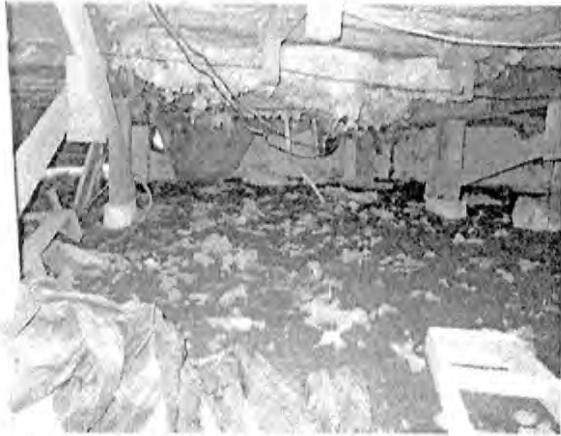
Timber-framing bears on a concrete wall and concrete piers beneath the church. The vapor barrier is incomplete.
