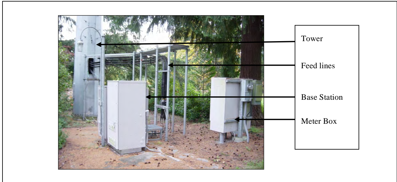
Figure 1: Example of 1900 MHz Wireless Infrastructure Ground Equipment
