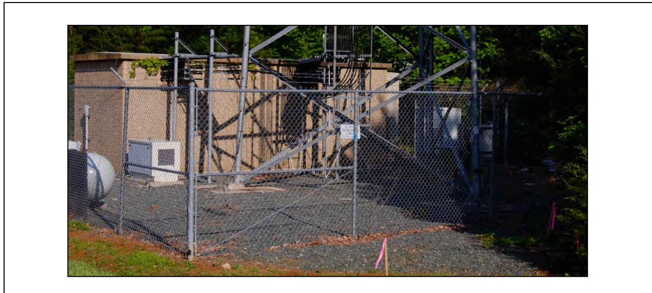
Figure 2: Example of 800 MHz Base Station
