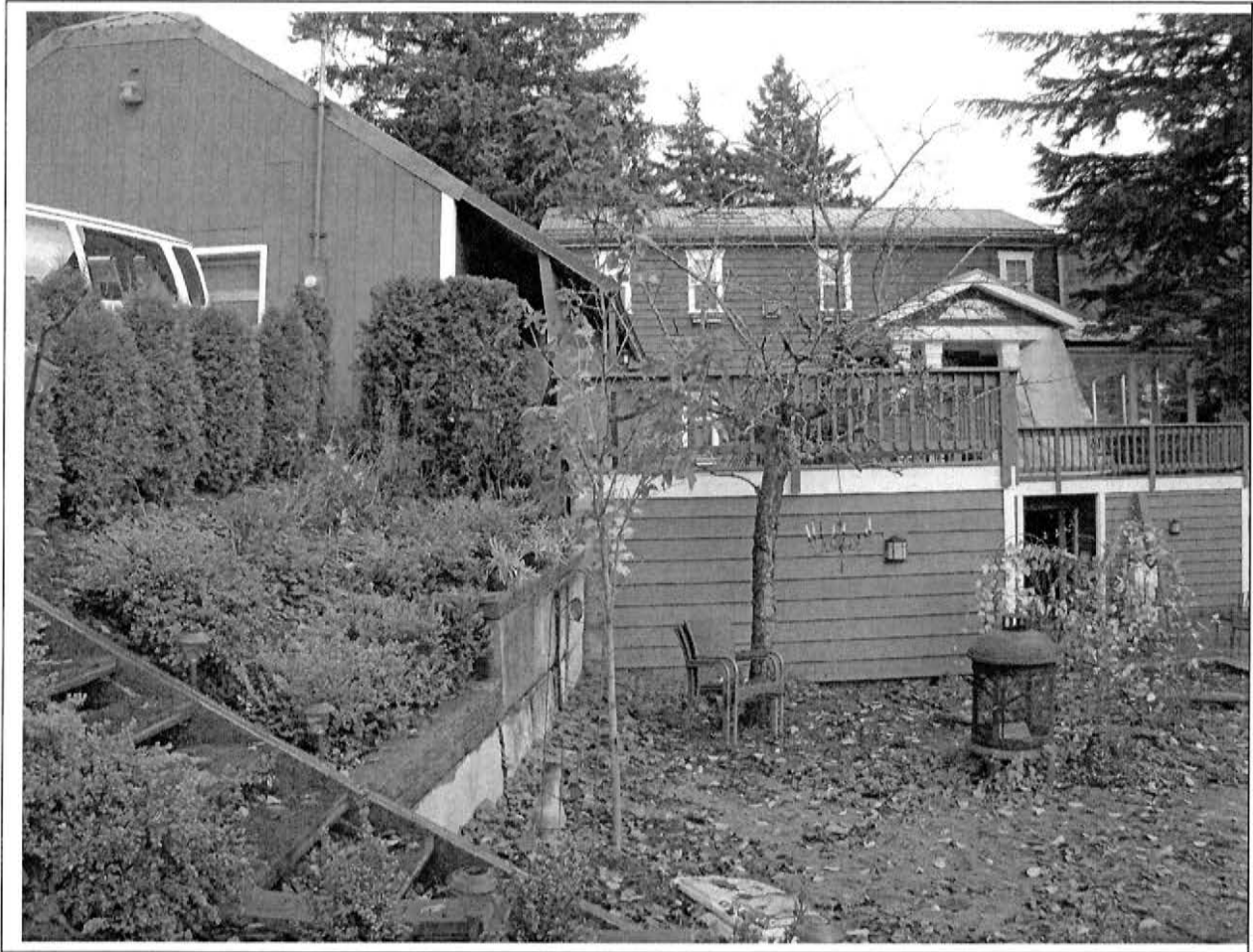
Figure 2: South side of garage from Spruce Street
