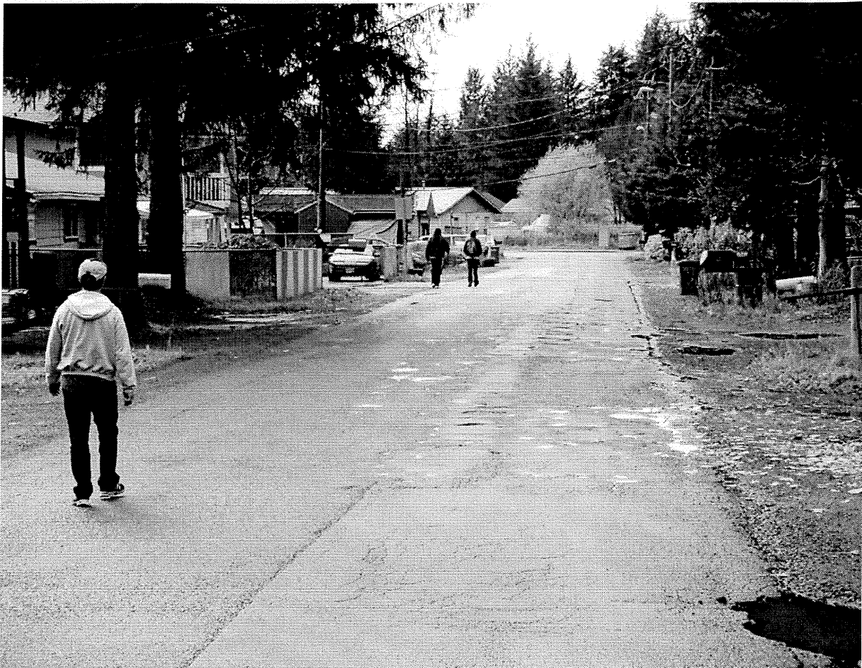
Figure 1: Lemon Creek Road facing west
