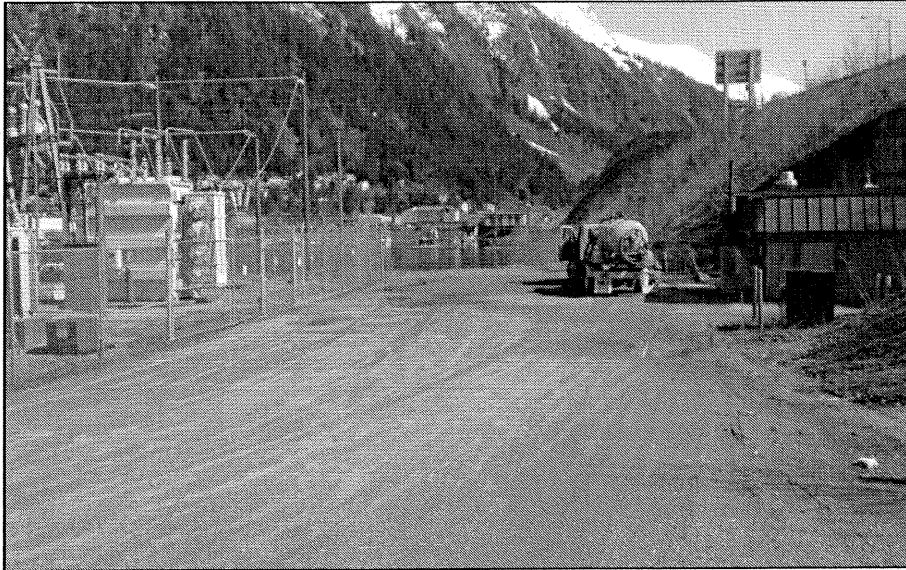
Figure 2: The Juneau-Douglas Bridge hillside is to the right side of the picture with the driving surface several stories above the electrical substation to the left. Picture taken by staff 4-29-13.
