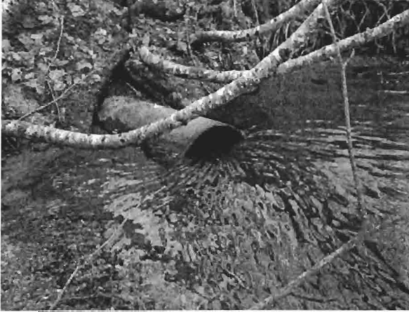
Figure 9. West berm culvert inlet at low tide.
