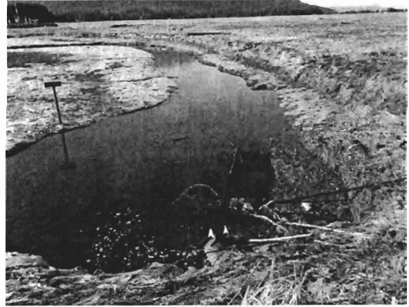
Figure 10. West berm culvert outlet at 1.8 m tide.
