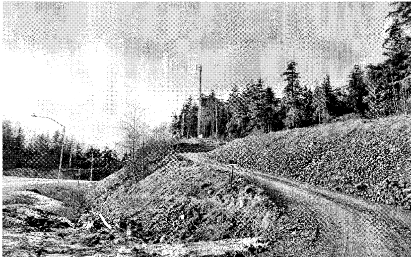
View of subject property looking in a westerly direction. Note 021812_0562 the other proposed 90' metal monopole to the right of the existing 75' wooden pole.
