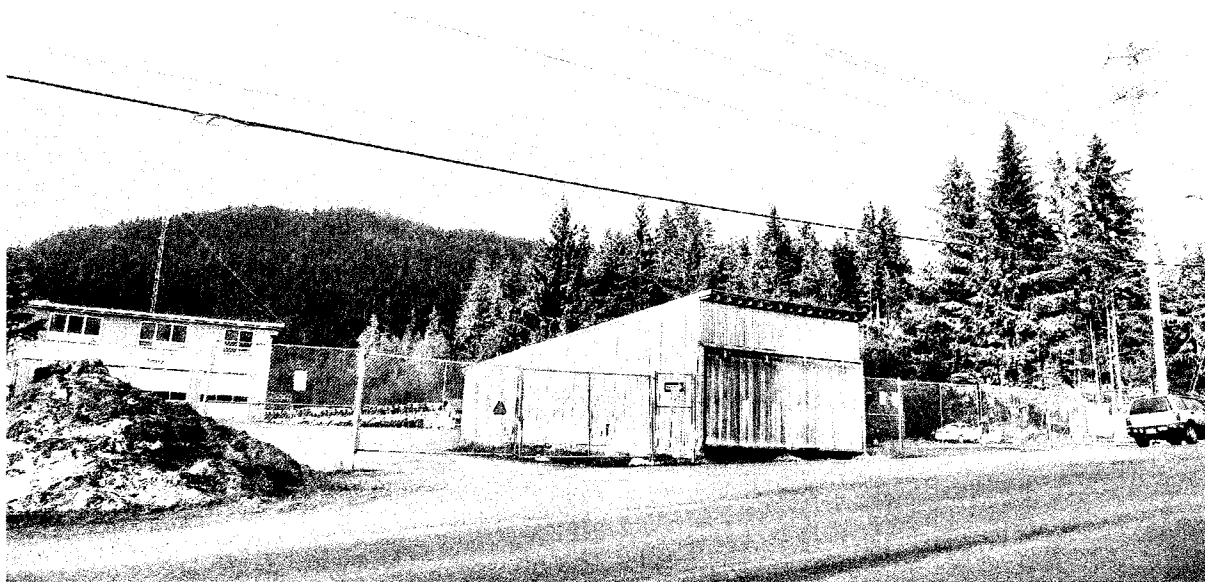
Proposed 150' tower would be 500' beyond the fence behind the building photo left. Existing 100' tower photo right. 021812_0559
