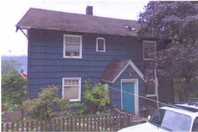
Mead Apts. (photo: Google Street View)
