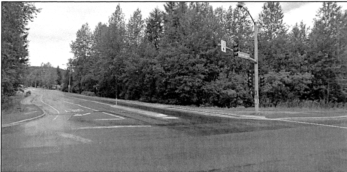
Figure 1: Picture of western end of Stephen Richards Memorial Drive intersecting Mendenhall Loop Road. Narrow island in road will be removed and the right traffic light pole and curb will be pushed back towards the woods to accommodate a new left-hand turn lane. Picture provided by Google Street View, dated 2010.
