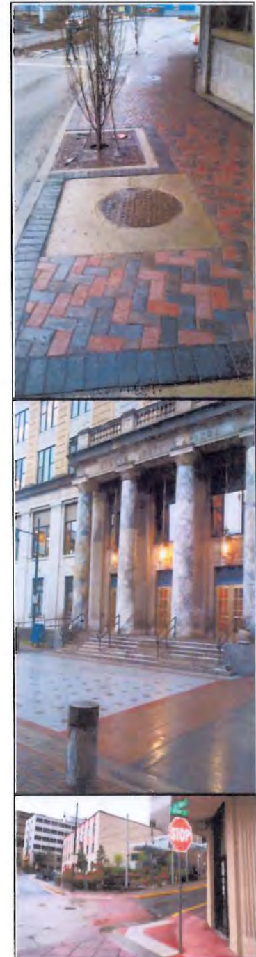
Colored concrete and brick, patterns, and attention to design all make crossings visible and signal that this is a special place. (from top: Main St sidewalks by new parking garage, crossing by Capitol, and Seward St intersection)
