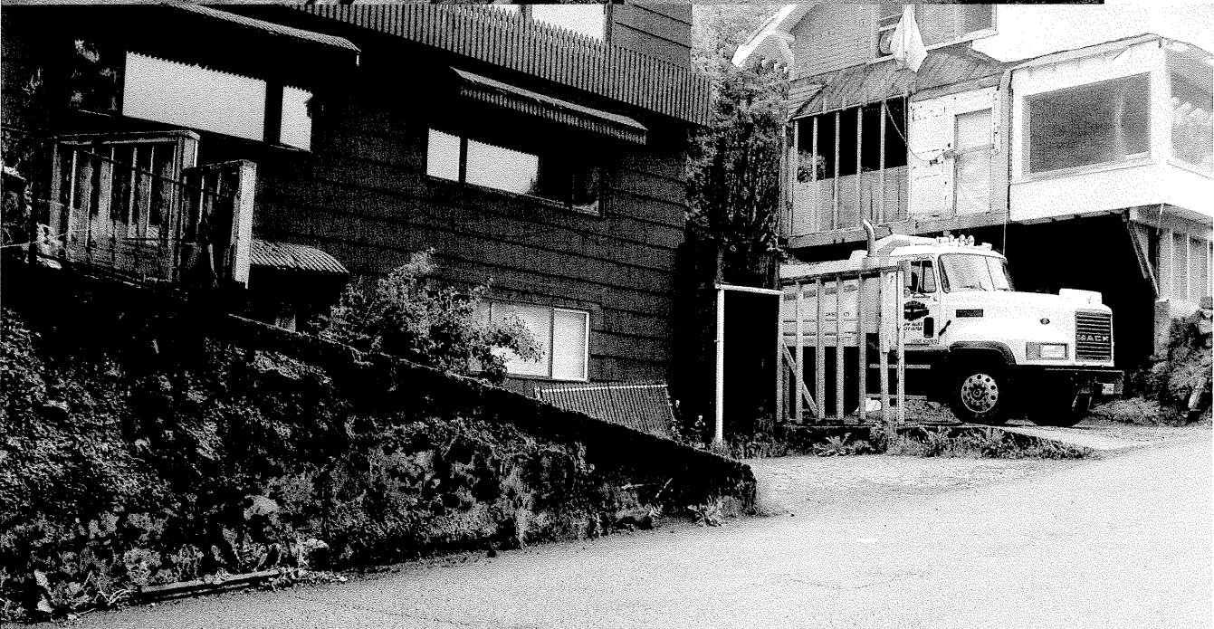
Photo taken 7/5/2011 - After demo and site prep for foundation began.
